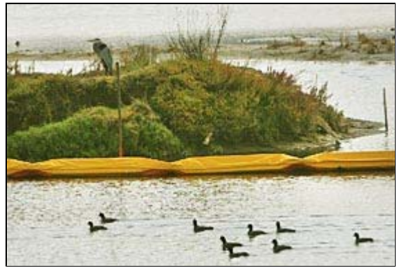
DON KOHLBAUER / Union-Tribune Even as heavy equipment rumbles about, several species of birds have checked out the habitat and found it to their liking. Five nesting sites are being built around San Dieguito Lagoon for endangered and threatened waterfowl.
