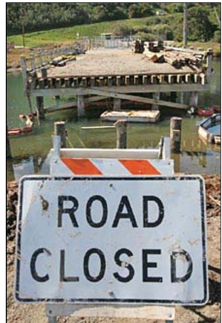
DON KOHLBAUER / Union-Tribune The Grand Avenue bridge will be kept and used as a viewing area near Del Mar Fairgrounds. Several viewing platforms are planned for the preserve.
